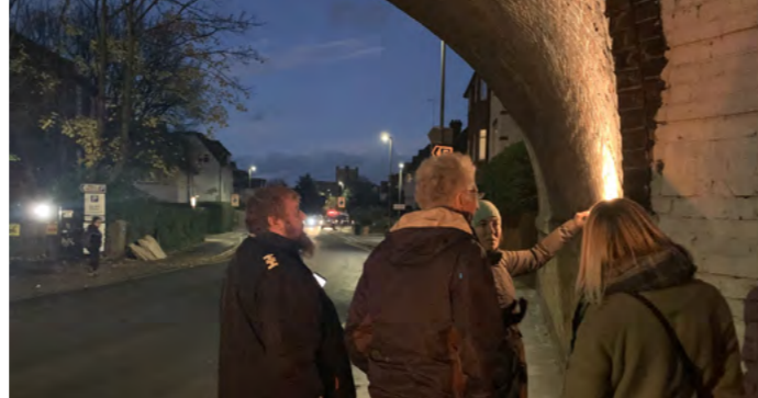
Hope Lane railway bridge. This bridge with the special diagonal brickwork could be highlighted. Could become point of reference and enrich the quality of the space around.
