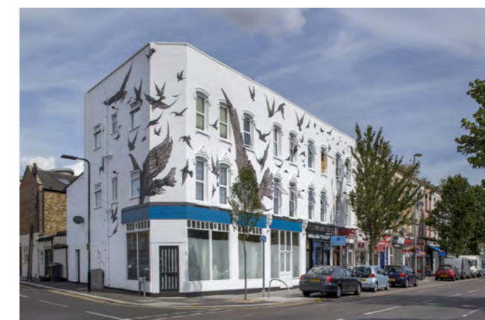
Jan Kattein Architects with MJO Signwriting mural after Alfred Hitchcock's 'The Birds.'
