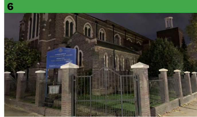
6 Greek Orthodox Cathedral. No exterior lighting creates a dark area by the high street and opposite the library.
